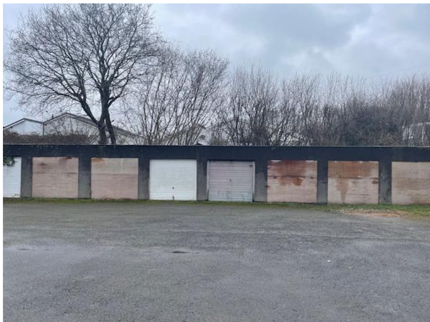
FIGURE 12: GARAGES TO BE DEMOLISHED
